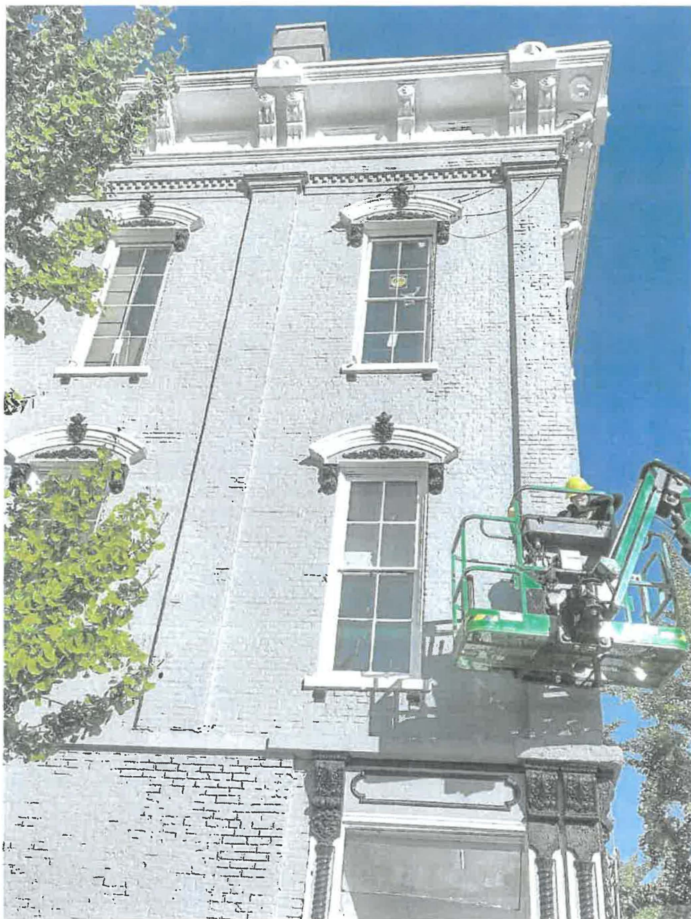
Picture A- The top right window has the added meeting rail.
